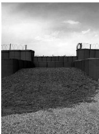
"Mounted fighting positions are designed to drive a Humvee into place."
